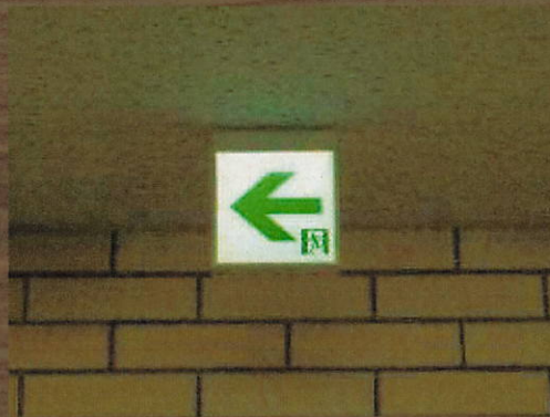
避難通路誘導灯
